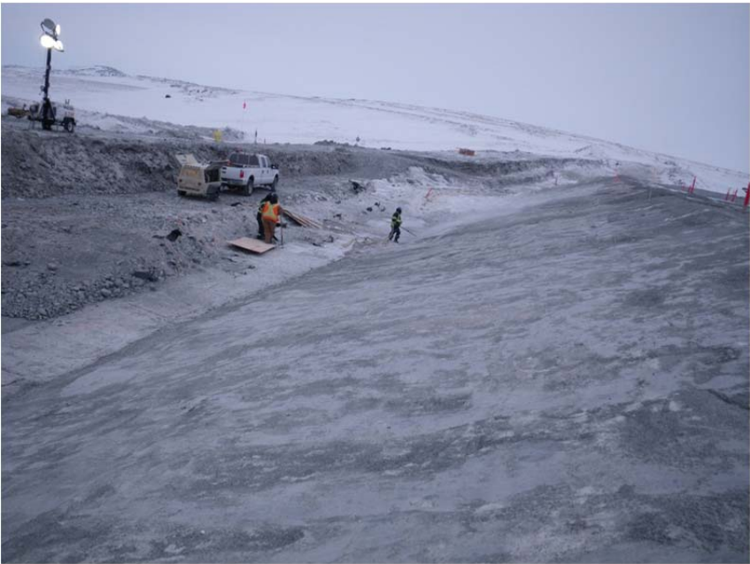
Photo 4: Looking south west along the upstream slope of the core. Labourers using air compressor to clean the slope.
