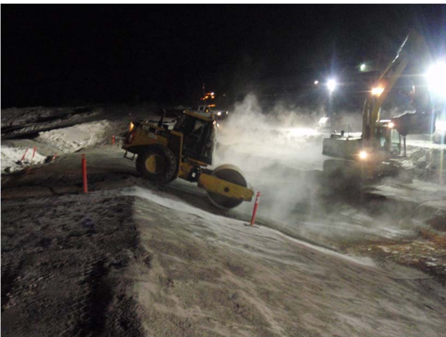
Photo 12: Packer working from the top to the bottom of the slope during Overliner placement.
