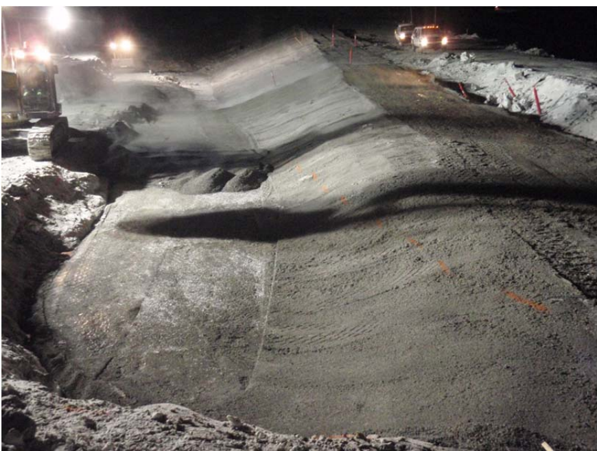
Photo 11: View of second lift of Overliner material starting to be placed at the N end of the core.
