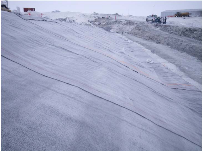
Photo 6: View of GCL placed along upstream slope of core. Photo looking north east along dam.
