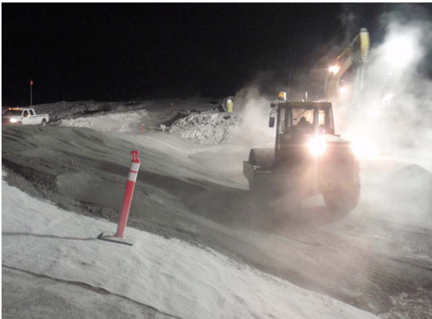
Photo 10: ~NEE view of Overliner material placement.
