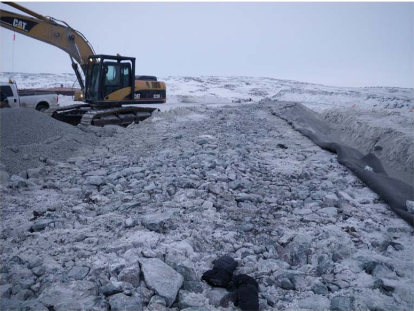
Photo 3: Looking south west at the ROQ along the top of the diversion berm. The ROQ surface does not appear packed; however this could be due to the excavator running on the packed surface.
