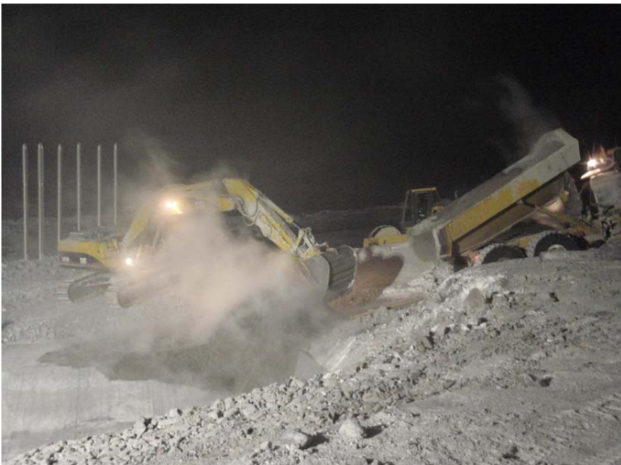
Photo 7: The start of Overliner GCL material placement (at ~ 1+95)
