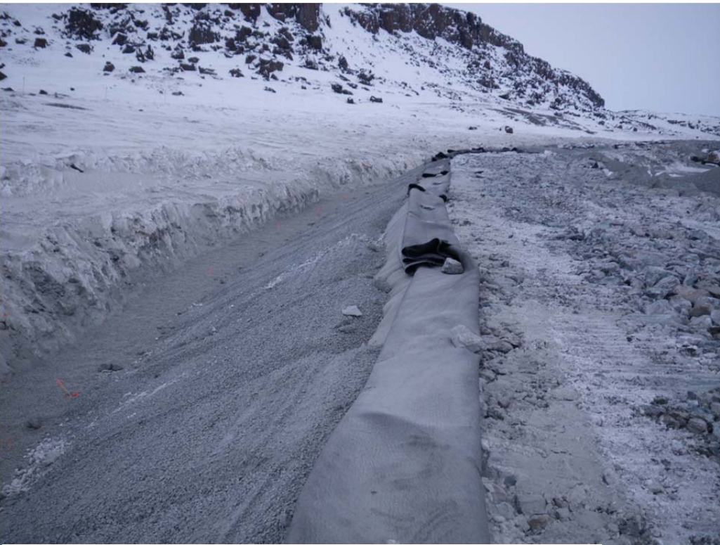
Photo 5: Underliner crush placed on diversion berm. Photo looking east.
