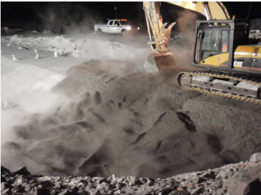
Photo 8: Excavator spreading first few loads of Overliner material on the N end of the core.
